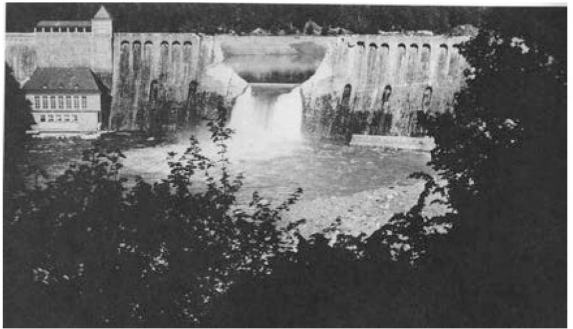
The Eder Dam after the breach.
