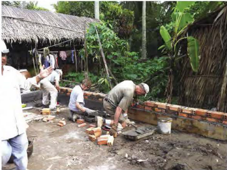
The walls go up.
