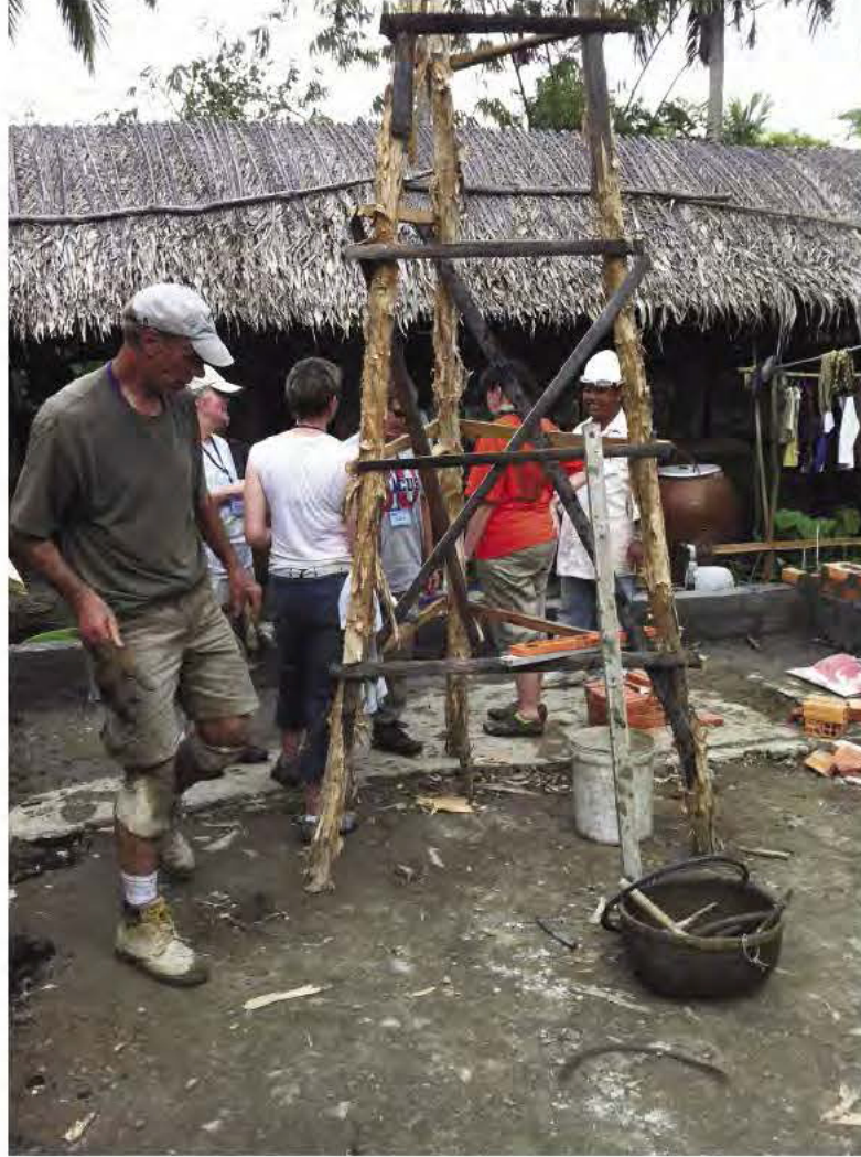
Building forms for the walls.
