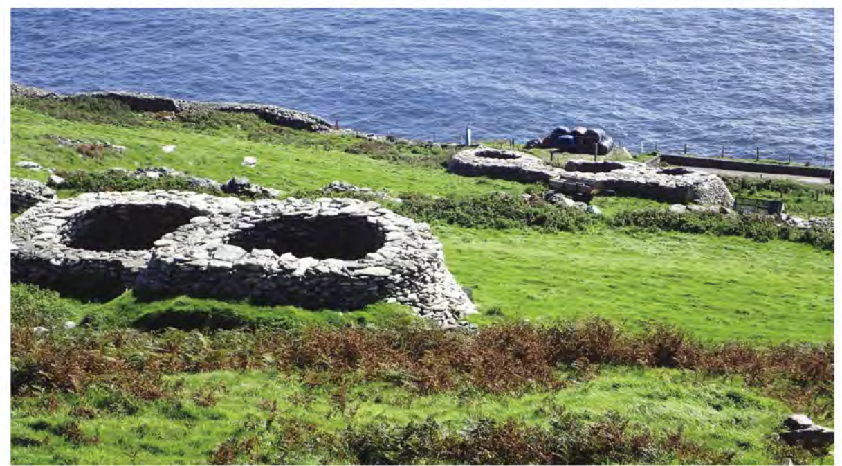
Beehive Huts, Clochans, built in circular layers, each with a smaller diameter than the one below.
