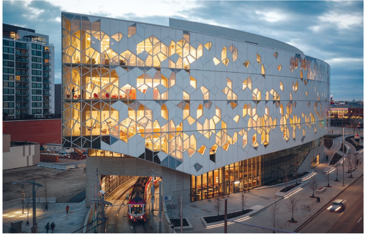
Calgary C-Train runs under the new Central Library.
